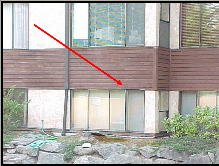
Siding was removed in multiple locations for inspection of the building paper, flashing details, and sheathing.
